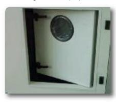
and hinges, or closing latches, according to the requirements and specific possibilities of the application. The accessible areas in negative pressure will have outwards-opening doors – the accessible areas operating under positive pressures will have inwards-opening doors. In compliance with the CE 89/392 Machine Directive, related to the safety in motor-fan sections, a counter-door is installed behind the fan access door, named 'anti-accident grid' with the same
